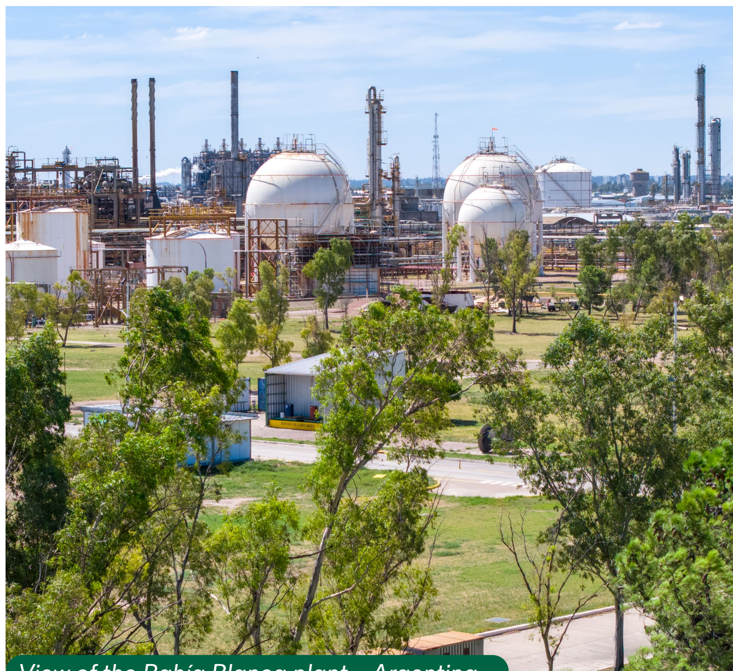
View of the Bahía Blanca plant – Argentina
