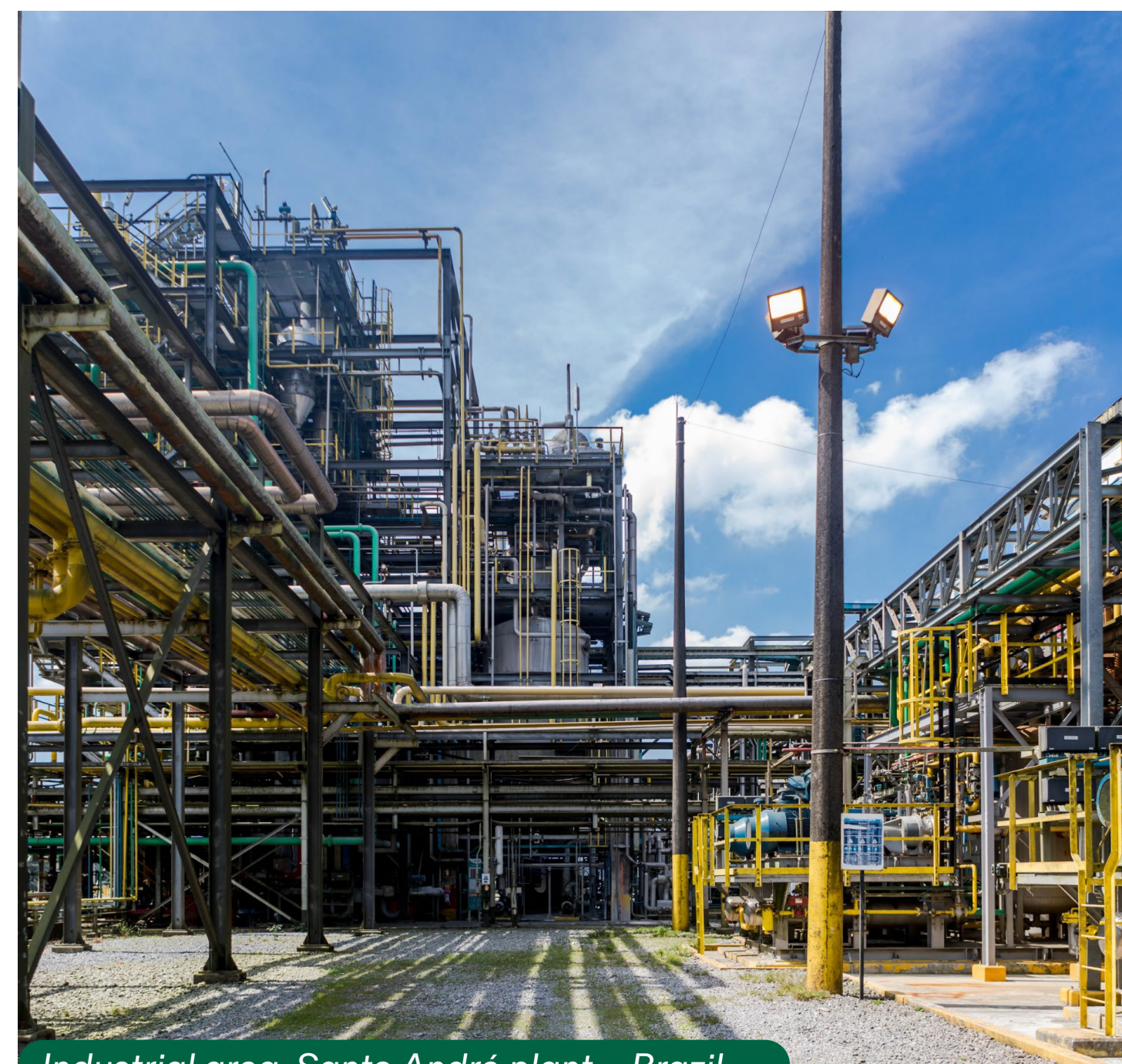
Industrial area, Santo André plant – Brazil
