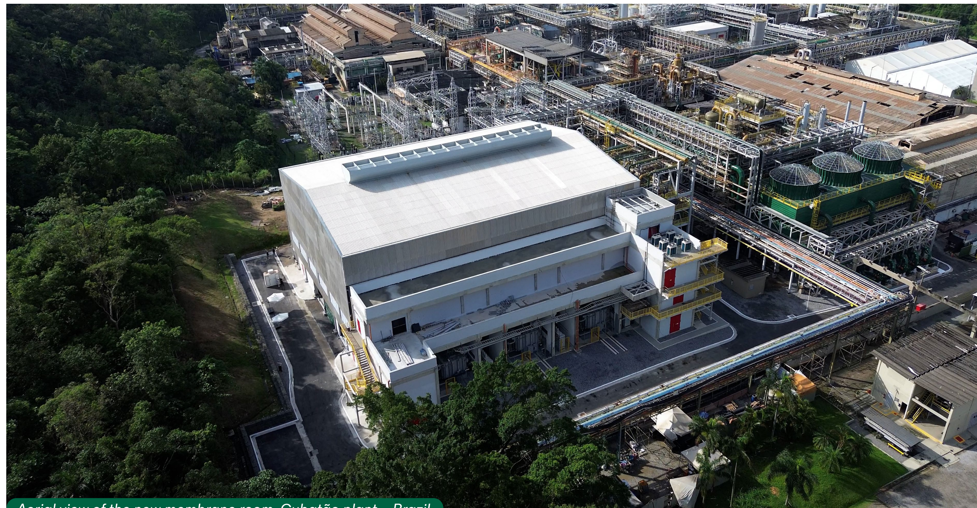
Aerial view of the new membrane room, Cubatão plant – Brazil
