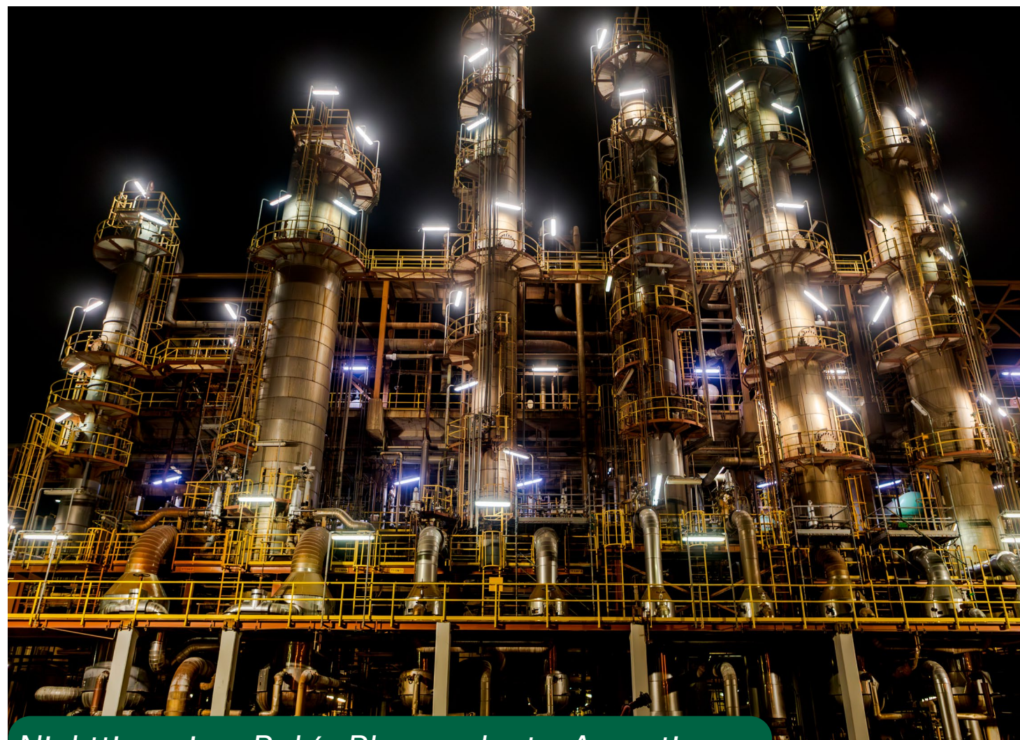
Nighttime view, Bahia Blanca plant – Argentina
