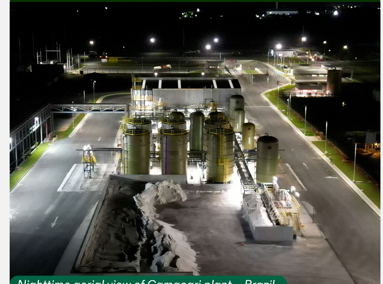
Nighttime aerial view of Camaçari plant – Brazil
